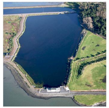
The distribution channel conveys treated wastewater into the intertidal storage basin where it is then discharged via the pump station.
